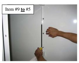
Position 3<sup>rd</sup> compartment ceiling and loosely attach a few 1/4" x 3/4" hex head bolts and washers where 3<sup>rd</sup> compartment divider and ceiling meet with rear passenger-side ceiling. This is the most difficult section to install due to aligning all 3 materials. *Be sure to do this step prior to attaching any part of ceilings or 3<sup>rd</sup> compartment divider.*
